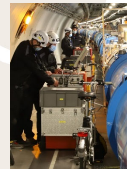
QC for interconnections of LHC magnets
