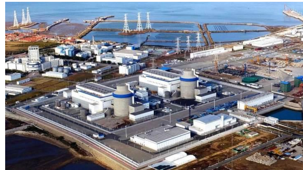
AP1000 reactors at Haiyang NPP, China
