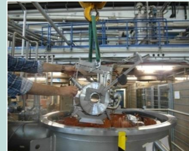
Magnet with CL installation in cryostat
