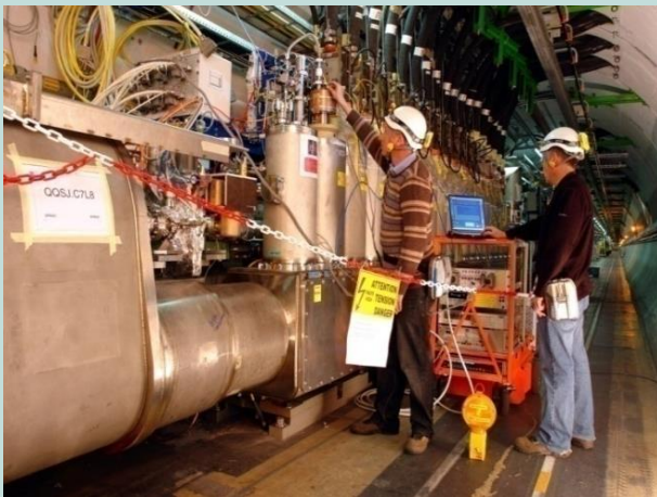
Mobil test stations in LHC tunnel
