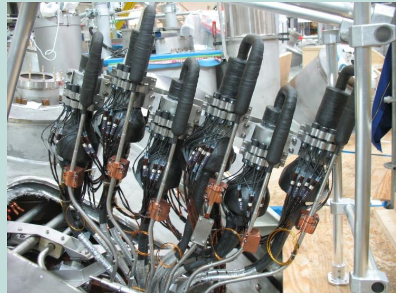
Module Separation Plane set of six joints painted and clamped
