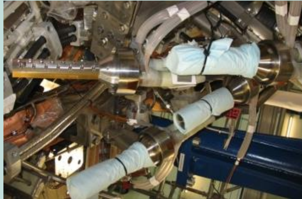
Connected triplets squeezed with clamps and covered by stainless steel caps
