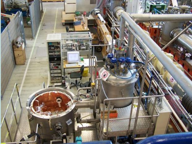
Hall 55 with cryogenic infrastructure for magnet tests
