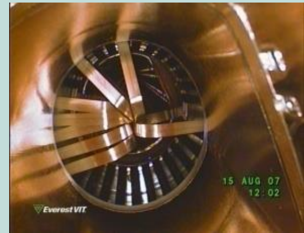
Damaged PIM ( Plug-In Module )
