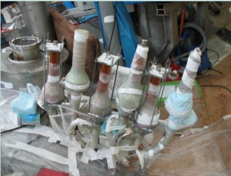
Installation of 24 bus bars on the module and final shaping of the bus bar ends
