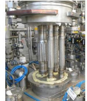
Installation of the XATL1 included precise positioning, high-quality welding works, wrapping superinsulations in the 16 module interconnections
