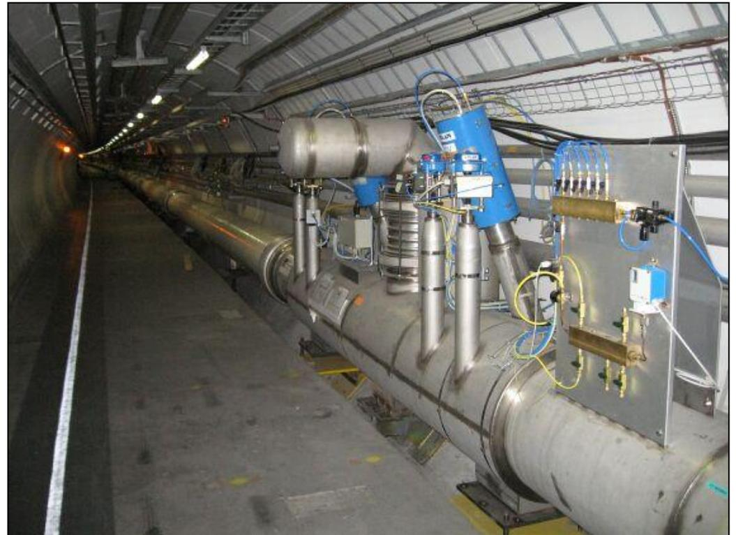
The LHC Cryogenic Distribution Line during the reception tests in sector 8-1
