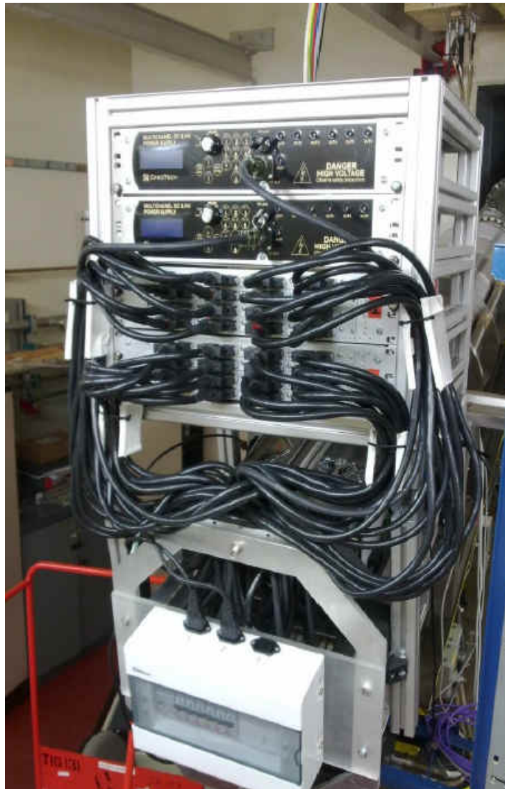
2 GEM system installation
