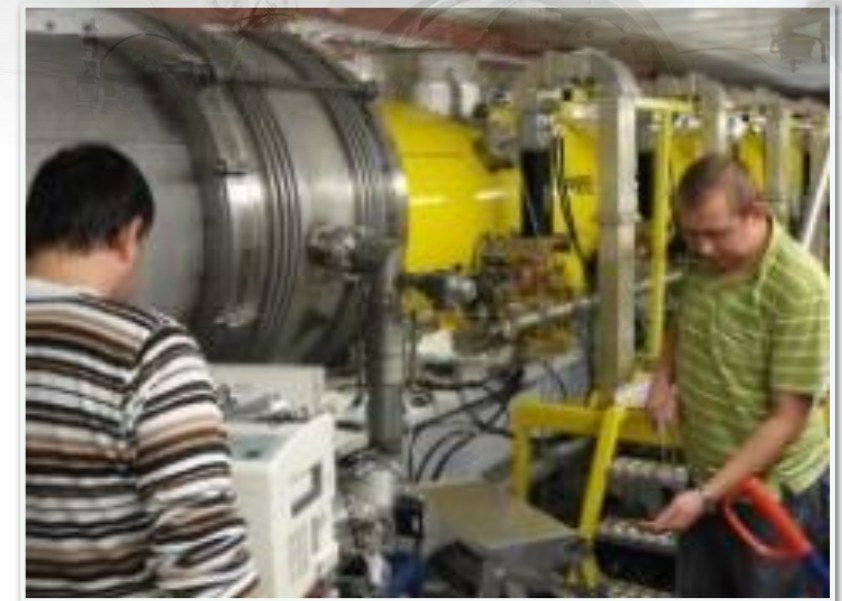
Leak test of vacuum pipes
