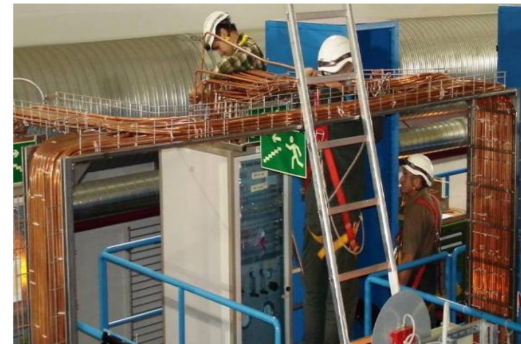
Muon Barrel piping
