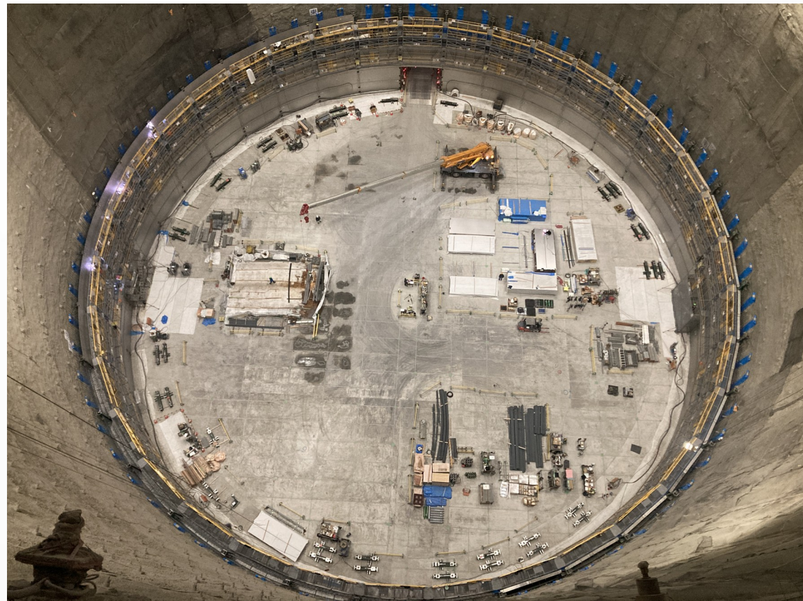
The barrel section of the main cavern, January 2026
