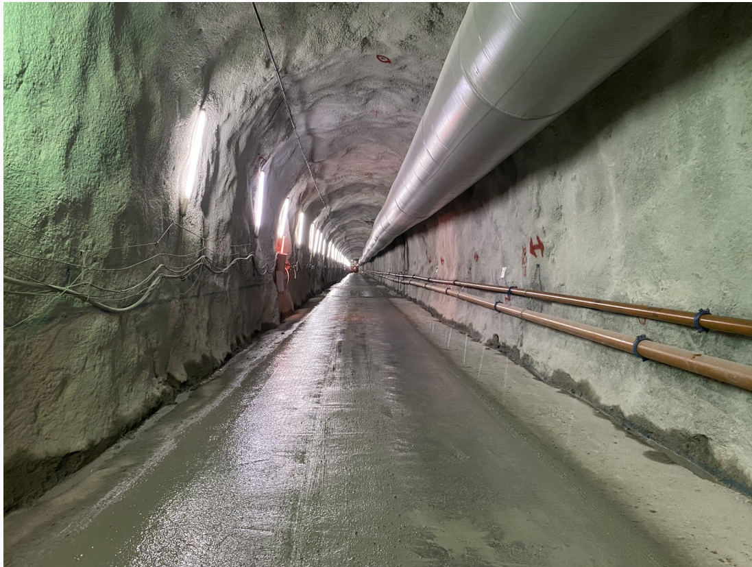
Paved part of the access tunnel, January 2022
