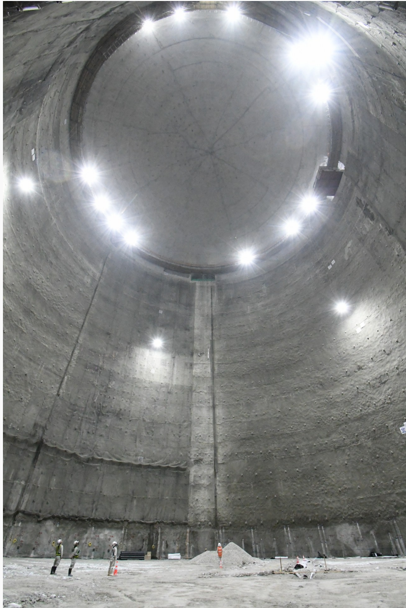
The main cavern completed, July 2025
