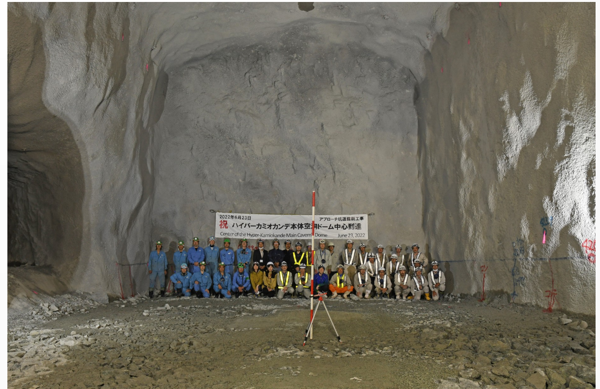
Center of the future Hyper-K Main Cavern's Dome reached, June 2022
