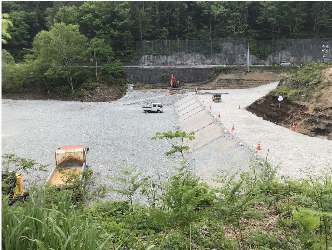
Entrance yard under construction, May 2020
