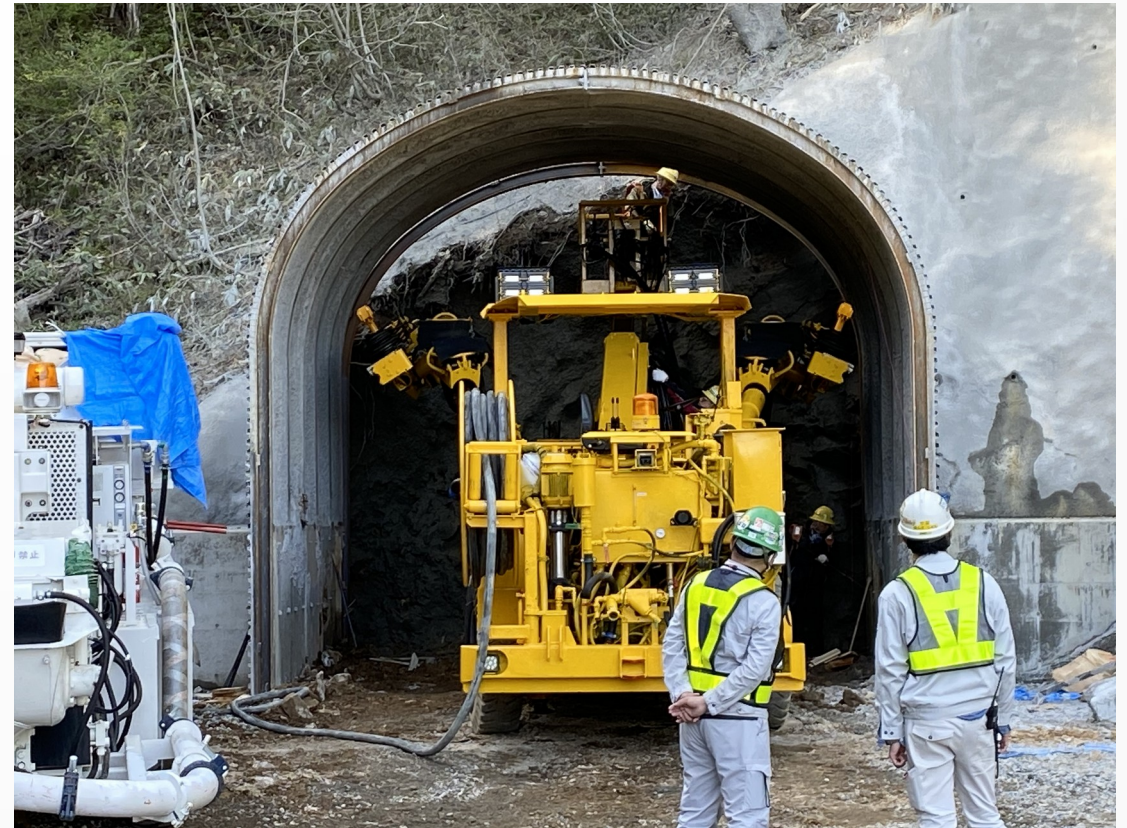
Excavation of the entrance tunnel, May 2021
