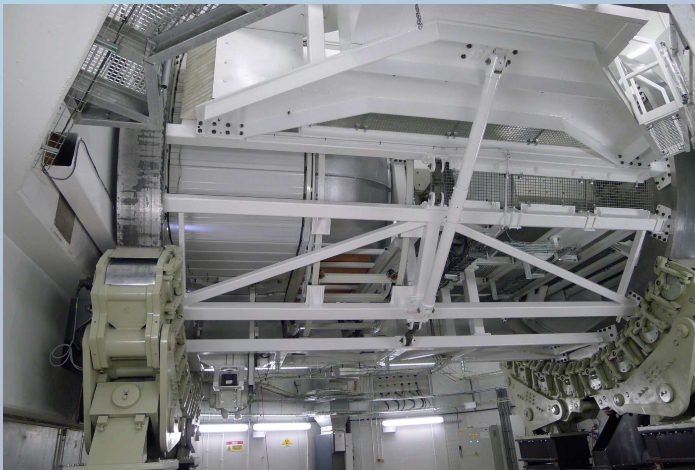
Gantry – side view
