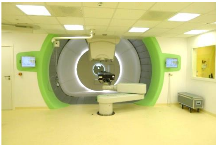
Two scanning gantries
